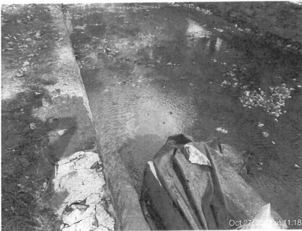
10/27/23 at 11:18AM. An opening at the end of the barrier allowed sediment to flow into the stream.
