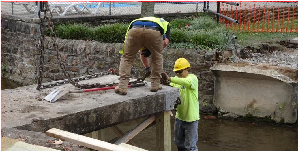
Chains from Excavator being Connected to Outer Edge to “Lever Up” and Pull Bridge
