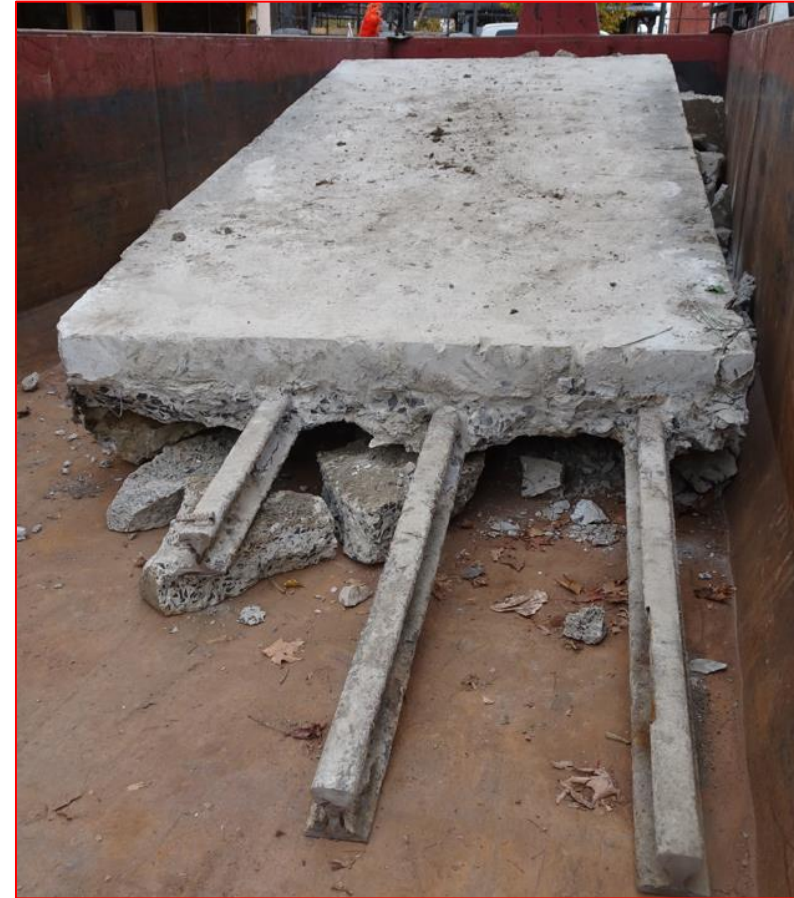
The Reason the Bridge was so Hard to Remove (Concrete Deck Strengthened by Internal Railroad Rails)
