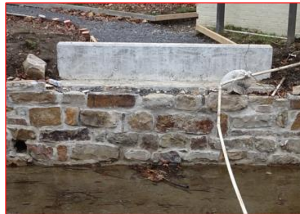
New West Side Abutment for New South Bridge (Behind new stone wall)
