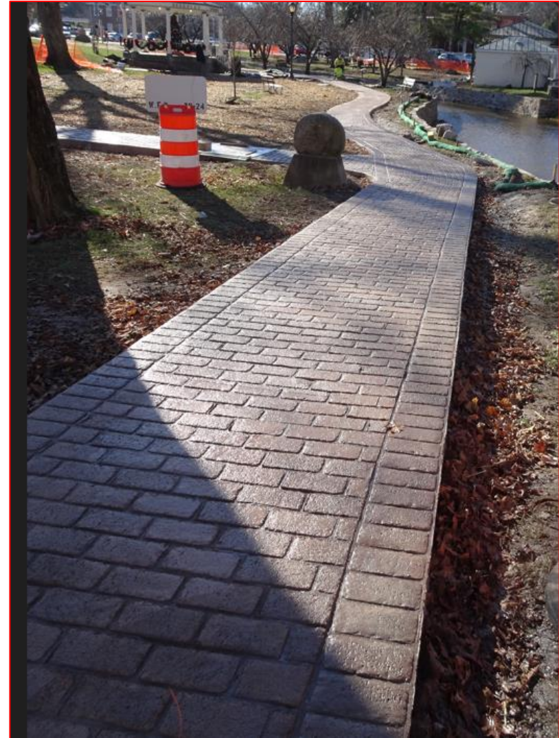
East of Run Sidewalk Looking South from Fairfax St (Section nearest camera is still wet (dark) from washing and sealant)
