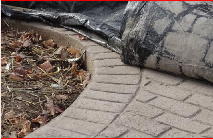
Example of Curved Area Edge Stamping at Sidewalk Intersection (Cleaning & Sealing not yet done)
