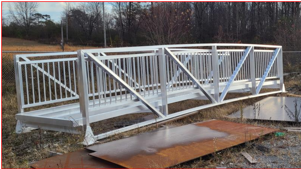
The New South Bridge at the Factory Prior to final Black Powder Coat and Decking
