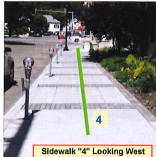
Sidewalk "4" Looking West adjacent to Court House
