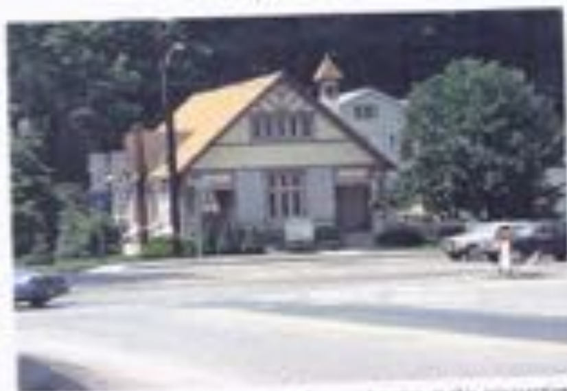
A traffic bottleneck and poor planning at this intersection.
