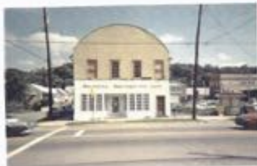
One of the few empty buildings detracts from the otherwise positive impression of downtown.
